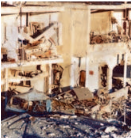
(3) Gulf War: Scud rocket attack on Israel on January 18, 1991: Damaged house in Tel Aviv.
